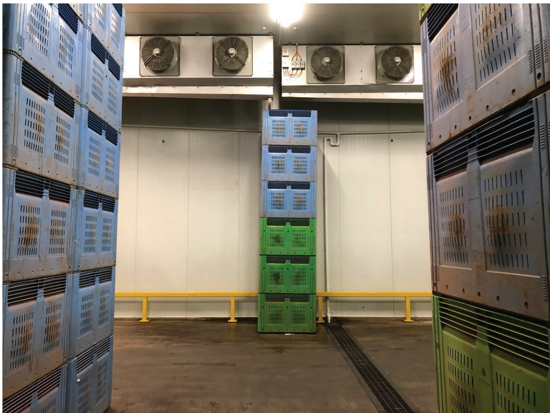
Figure 19. A pre-cooling facility in a melon packhouse.
